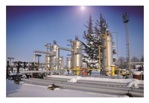
**Picture 2:** Whether in Alaska, Canada, Norway or Russia: Industrial valves as they are used are often exposed to extremely low environmental temperatures.
