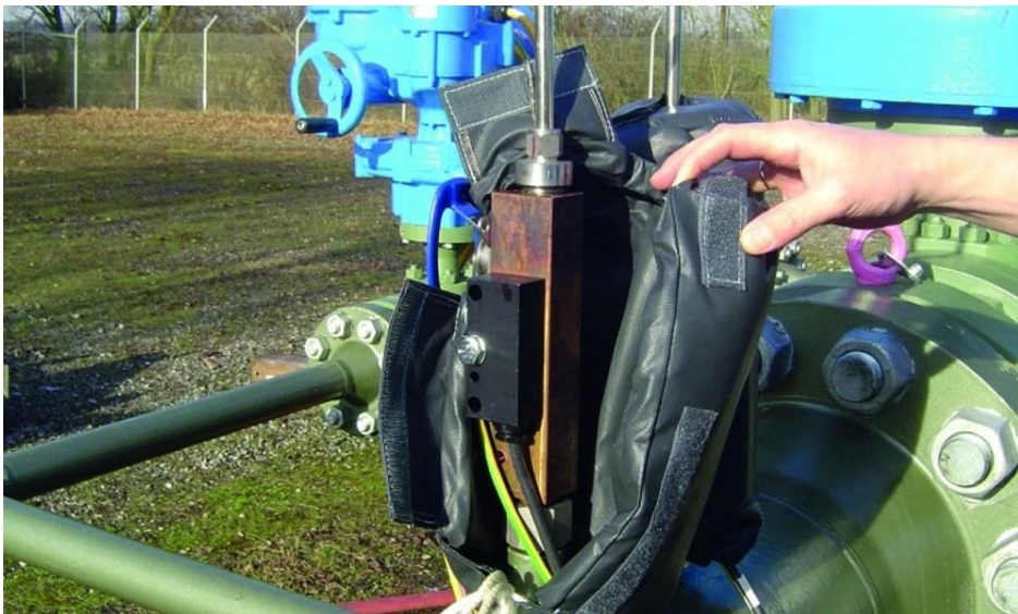
Picture 2: AS-Schneider has designed the heatable sampling probe to be compact. This makes it easy to install.
